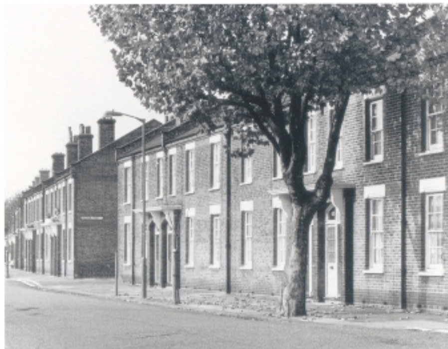
Upgraded sash windows fitted with draughtproofing in a South London terrace
