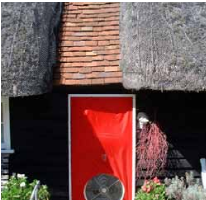
09 Pressure testing a timber framed building can give a good indication of where there is excessive air infiltration. Such areas can then be targeted in any planned thermal upgrading. © Oxley conservation
