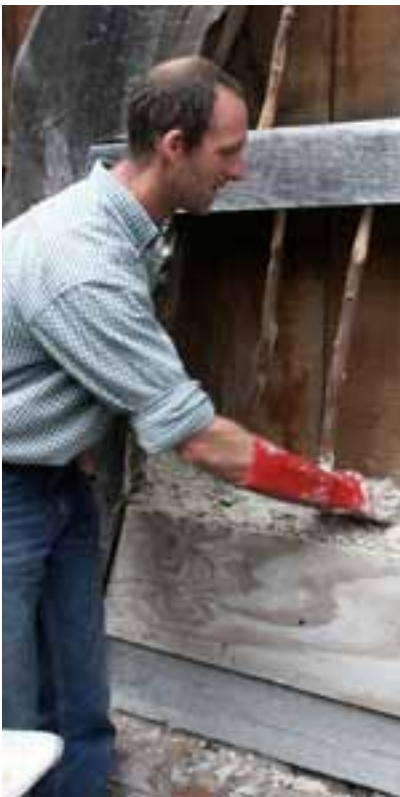
I0 Hemp-lime being installed as an infill panel. © EH/Iain McCaig
