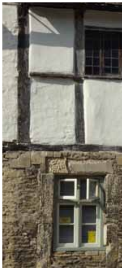
08 A timber frame above a stone ground floor. © EH/David Pickles
