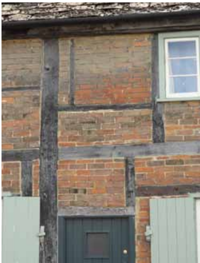
07 A timber framed cottage with brick infill panels. © EH/David Pickles
