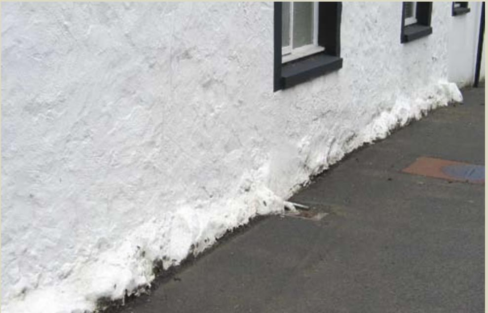
By Victorian times this protrusion had been regularised, and reduced in dimension, until only a minor thickening of the wall occurred at the footing. At the same time a more scientific approach emerged in designing foundations, resulting in the laying of proper load bearing strips upon which the building's walls were constructed.
