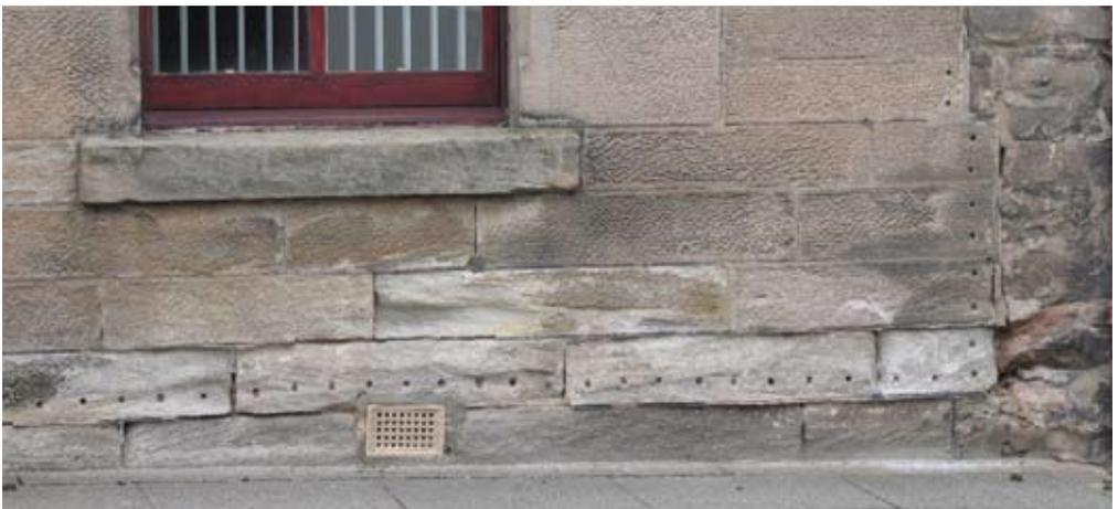
into the wall might include active and passive electro-osmotic techniques where electric currents are passed through the installed system in an attempt to control dampness.
