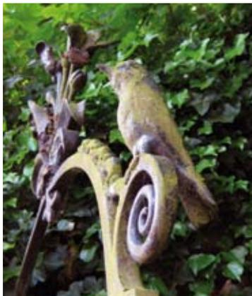
● New paint systems: Where the existing paint is in poor condition, it may be necessary to remove it entirely before repainting. However, if ironwork is listed or of special historical interest, the removal of original paint layers will need careful consideration and may merit further paint analysis to determine the original colour scheme that was used.
