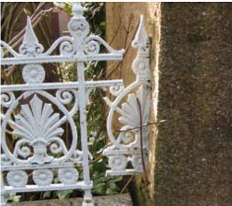
Fracturing can occur to stone where ironwork that has been fixed into masonry sockets corrodes and expands.
