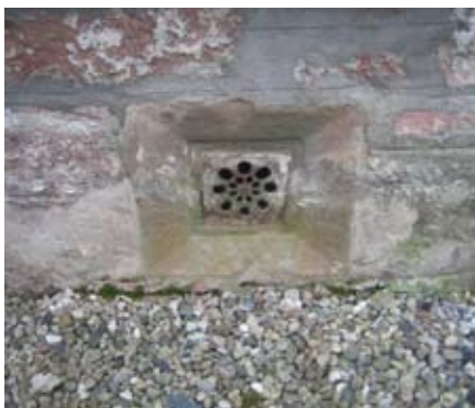
Ensure that external vents do not become blocked by rising ground levels around your property
