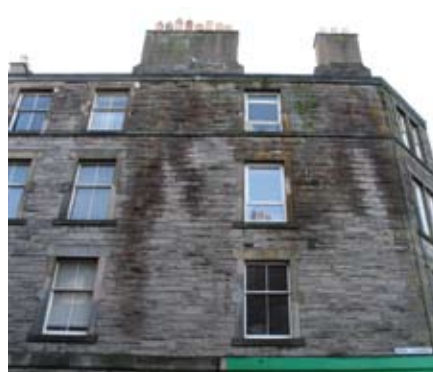
Damage to lead flashing and blocked rainwater goods can cause extensive damage
