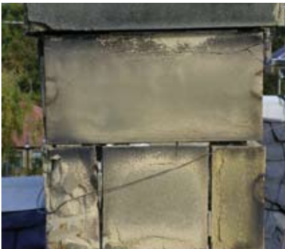
Check mortar pointing on chimneys especially around the pots and cans
