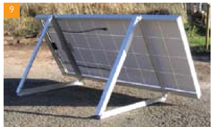
Ground-mounted PV array. (Photographs courtesy of Wind and Sun Ltd.)
