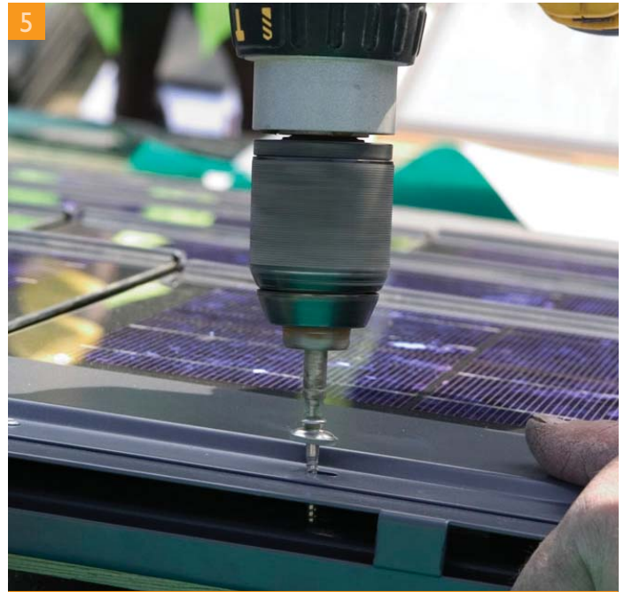
PV roof tile being drilled to timber roof batten. (Photograph courtesy of Solar Century)
