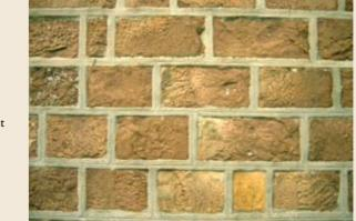
sound or resistant to removal it will be necessary to evaluate the likely damage that could be caused by leaving it in place against the damage which would be caused by its removal. Sometimes the best practical option is to leave the cement mortar in place, accept the existing appearance and, possibly, any ongoing related masonry decay.
