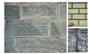
Water vapour egress through the lime mortar joints of ashlar masonry needs to be recognised as an important part of how traditional buildings breathe and cope with rain water. If this process is prevented from happening a number of damp related problems and consequences can emerge. The most common cause of such problems is the use of cement-based mortars to repoint the walling and this should be avoided in all repair work.
