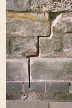
surfaces are dampened before pointing work starts. Any accidental spillage or smearing should be washed off immediately with a fine jet of clean water, but this could be avoided in the first place by setting some temporary protection in place below the work area to contain any spillage.
