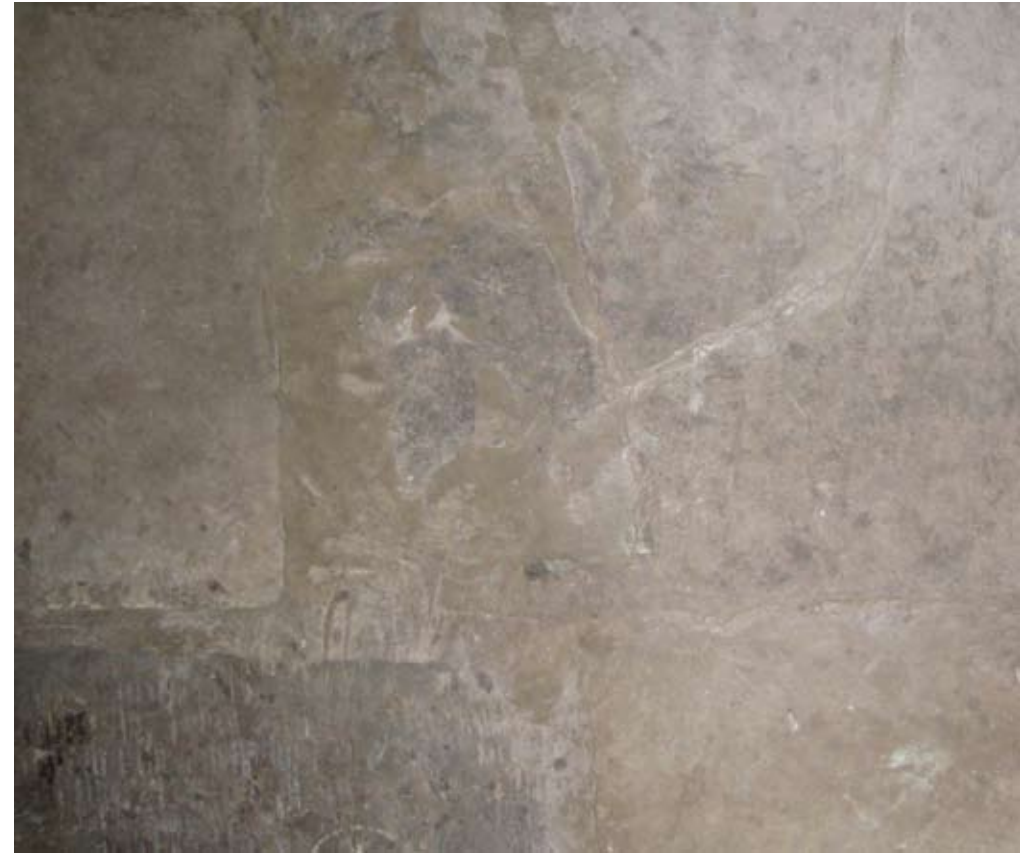
Historic impact damage showing subsequent repair
