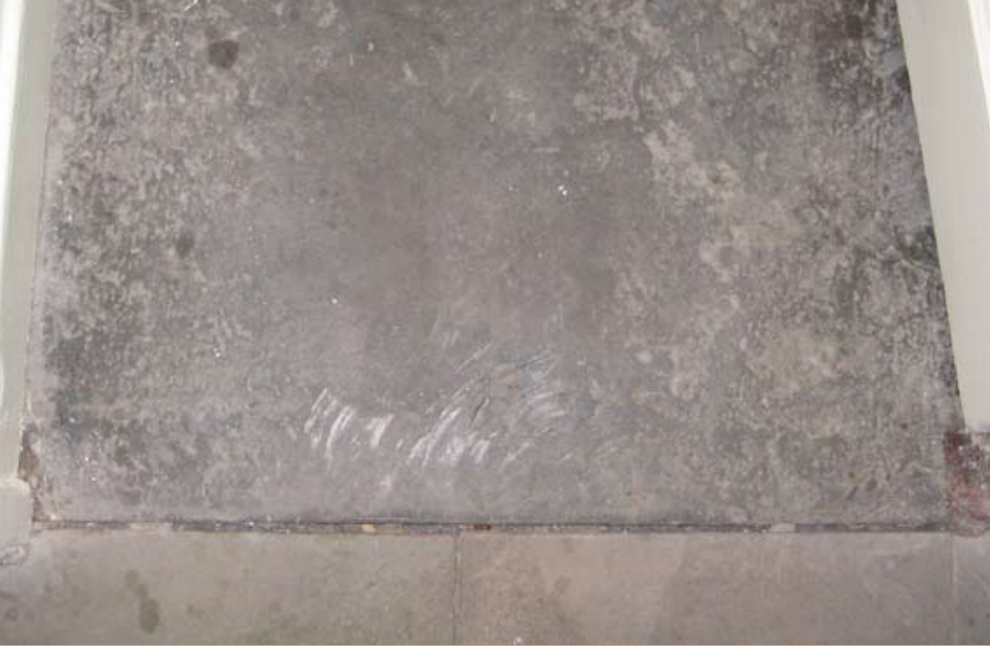
Repaired slab showing grinder marks and cement patching
