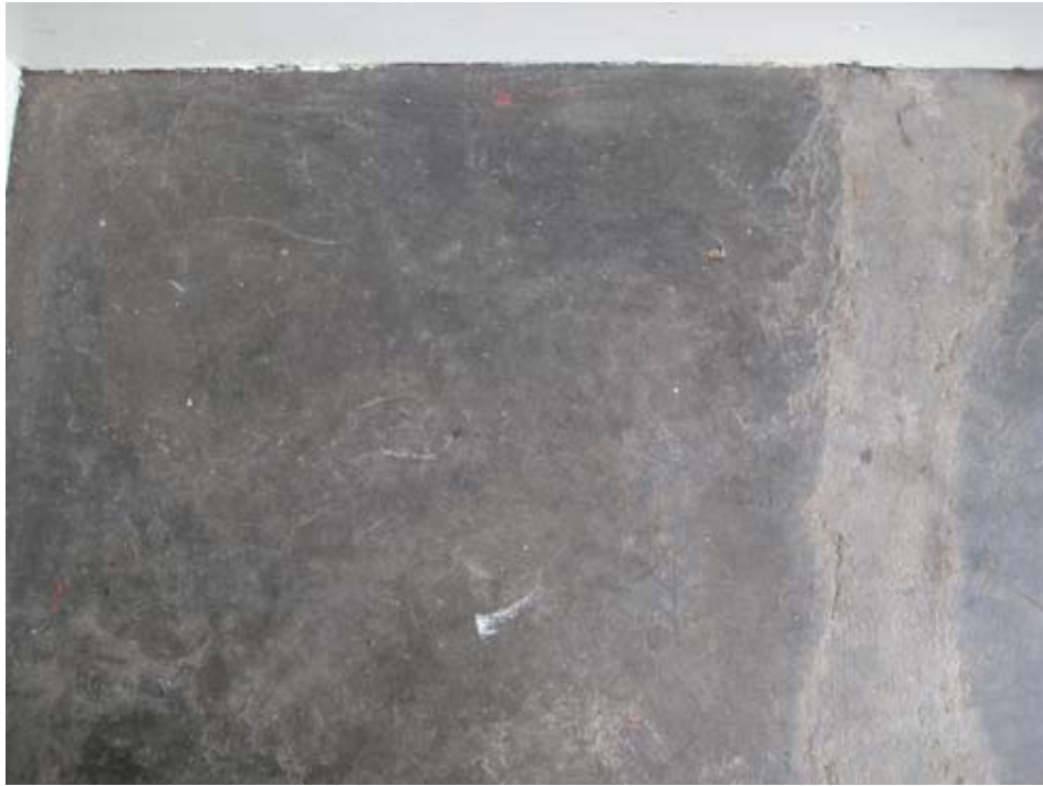
Carmylie slab sealed with linseed oil; note lime pointing to wide joint on upper side
