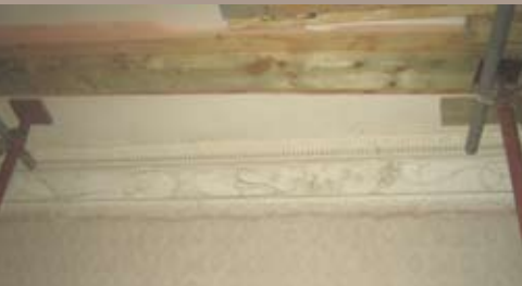
Supporting a ceiling during work on the joist ends
