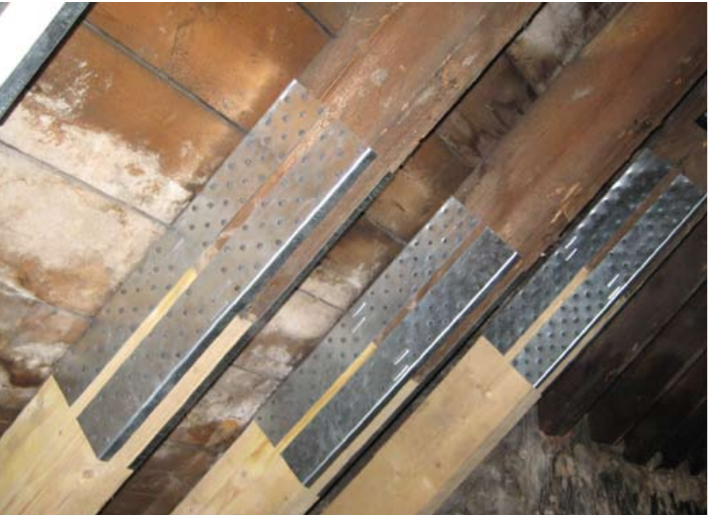
Modern metal pre drilled straps used in rafter splices.
