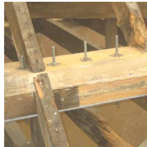
Composite repair using resin, new timber and steel plate
