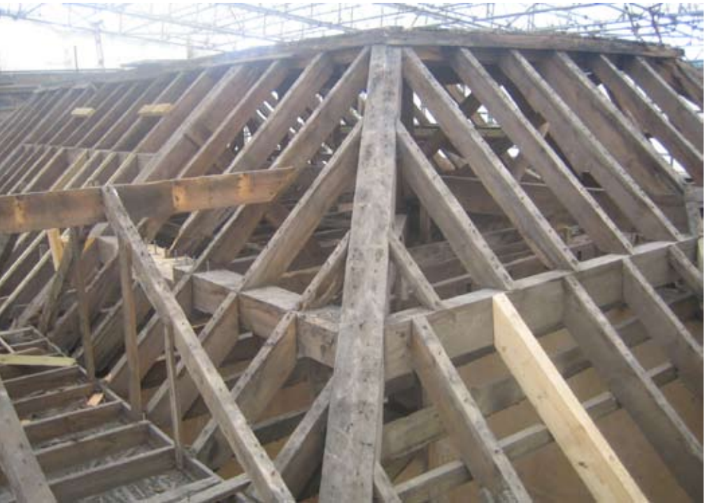
A roof of the Late 18th under repair, showing the purlins midway in the span.
