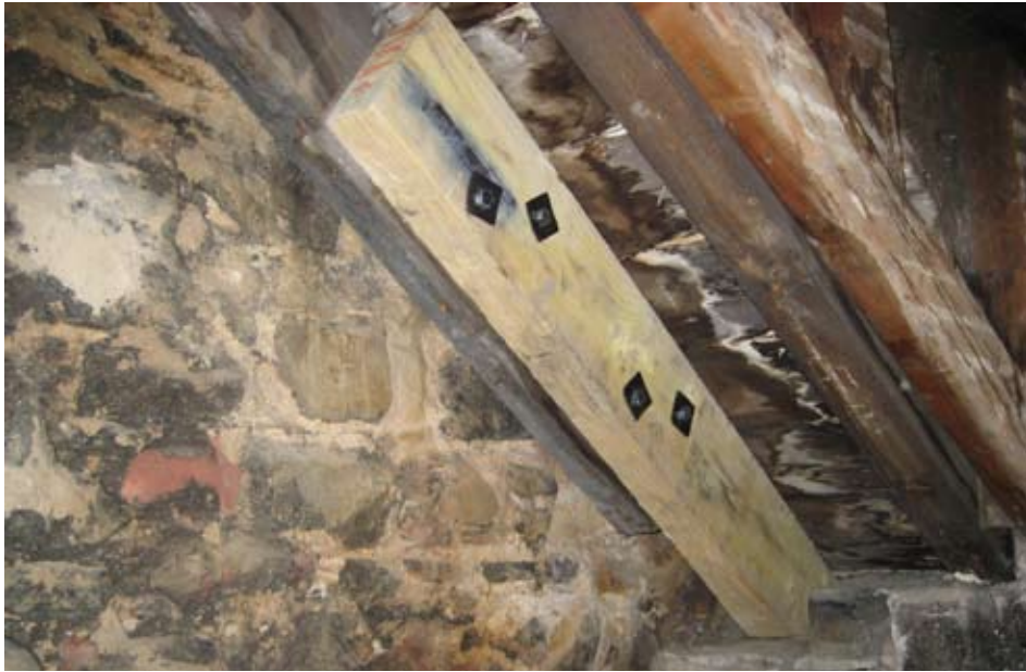
Strengthening of the joint with bolts
