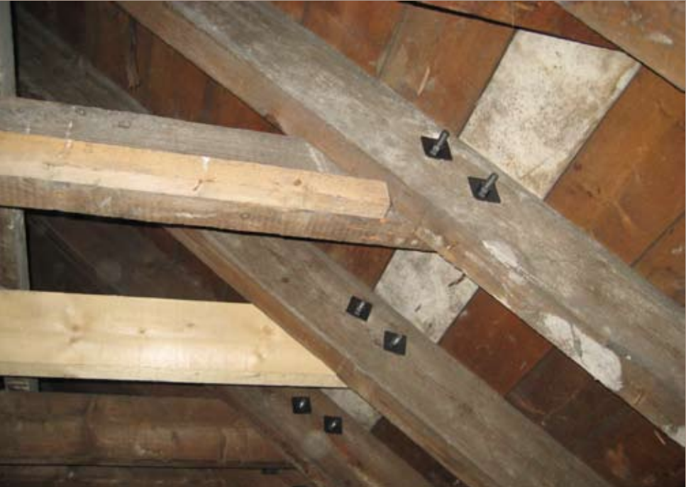
Strengthening of the joint with bolts
