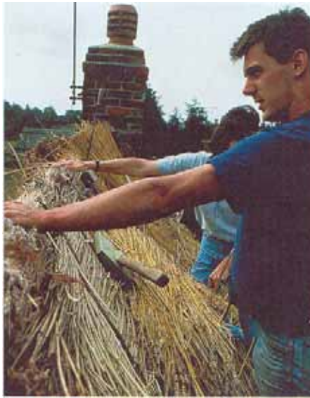
Fig 8 Forming the ridge during rethatching in combed wheat reed. The horizontal bundle used as a core for the ridge can be seen.
