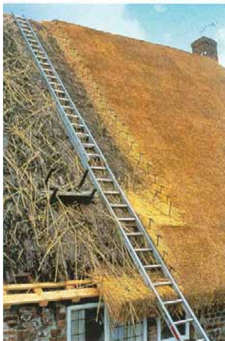
Fig 20 Combed wheat reed being sparred onto a pre-existing base of straw. This technique is also used to attach water reed to a straw base. (Photograph copyright © John B Letts)
