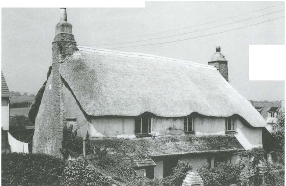
Fig 10 Combed wheat reed roof in Devon (late 1950s). (Photograph copyright @ Rural Development Commission)
