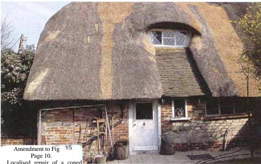
Fig 14 A mossy roof may look attractive, but usually indicates significant moisture retention. However, the moss may not be harmful.
