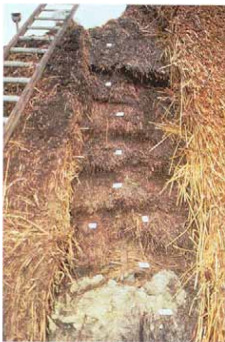
Fig 19 Stepped excavation of a roof showing the different identifiable layers. (Photograph copyright © John B Lens)
