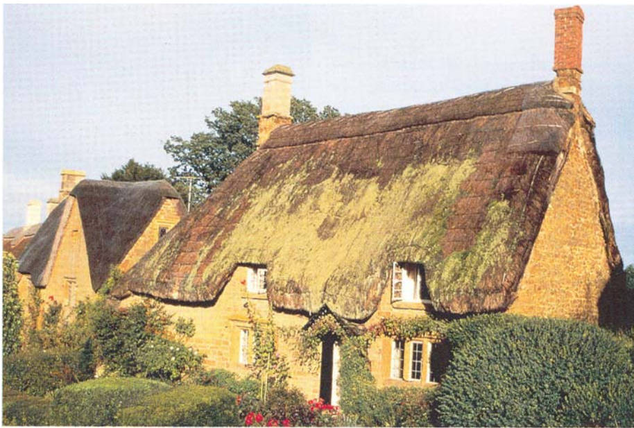
Fig 14 A mossy roof may look attractive, but usually indicates significant moisture retention. However, the moss may not be harmful.
