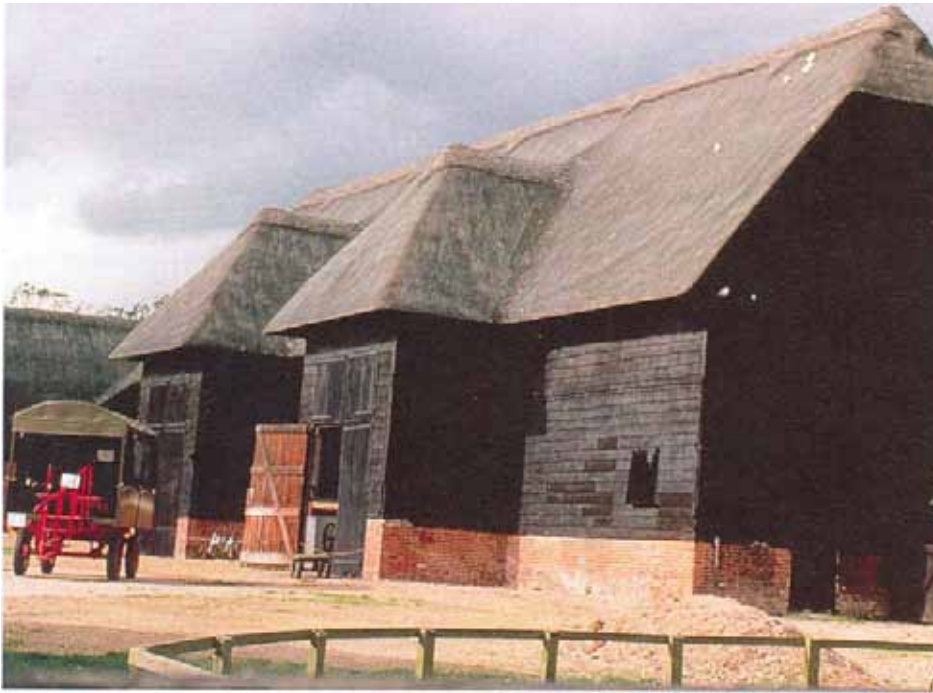
Fig 6 The great barn at Wimpole, Cambridgeshire, is thatched in water reed which faithfully follows the architectural structure under the thatch.
