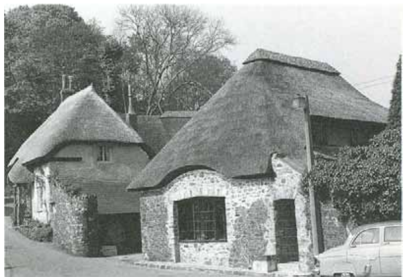
Fig 5 By contrast, the house in Devon (background) roofed in the same material, shows the more rounded outline of a typical hipped roof thatched in combed wheat reed. The house in the foreground is thatched in water reed. (Photograph copyright @ Rural Development Commission)
