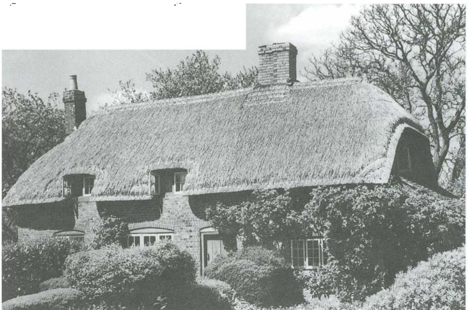
Fig 11 Long straw thatch in Hampshire, of the same date as Fig 10. (Photograph copyright @ Rural Development Commission)
