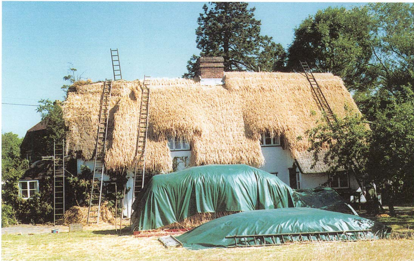
Fig 12 Thatching long straw to a basecoat
