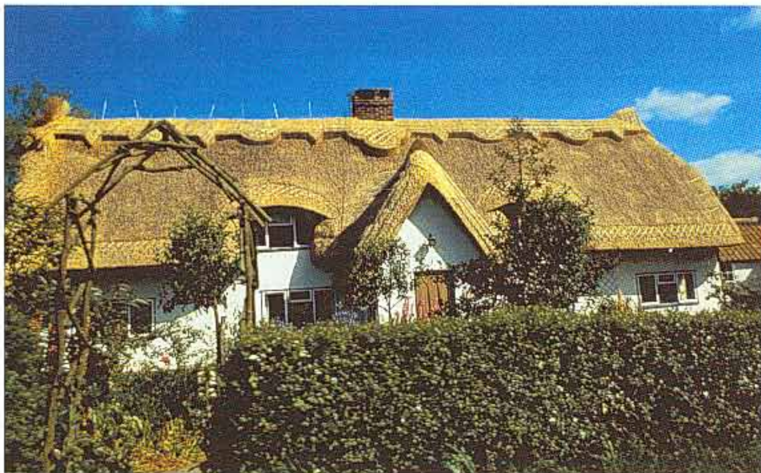
Fig 17 An elaborately patterned block ridge of the kind widely seen since the 1960s
