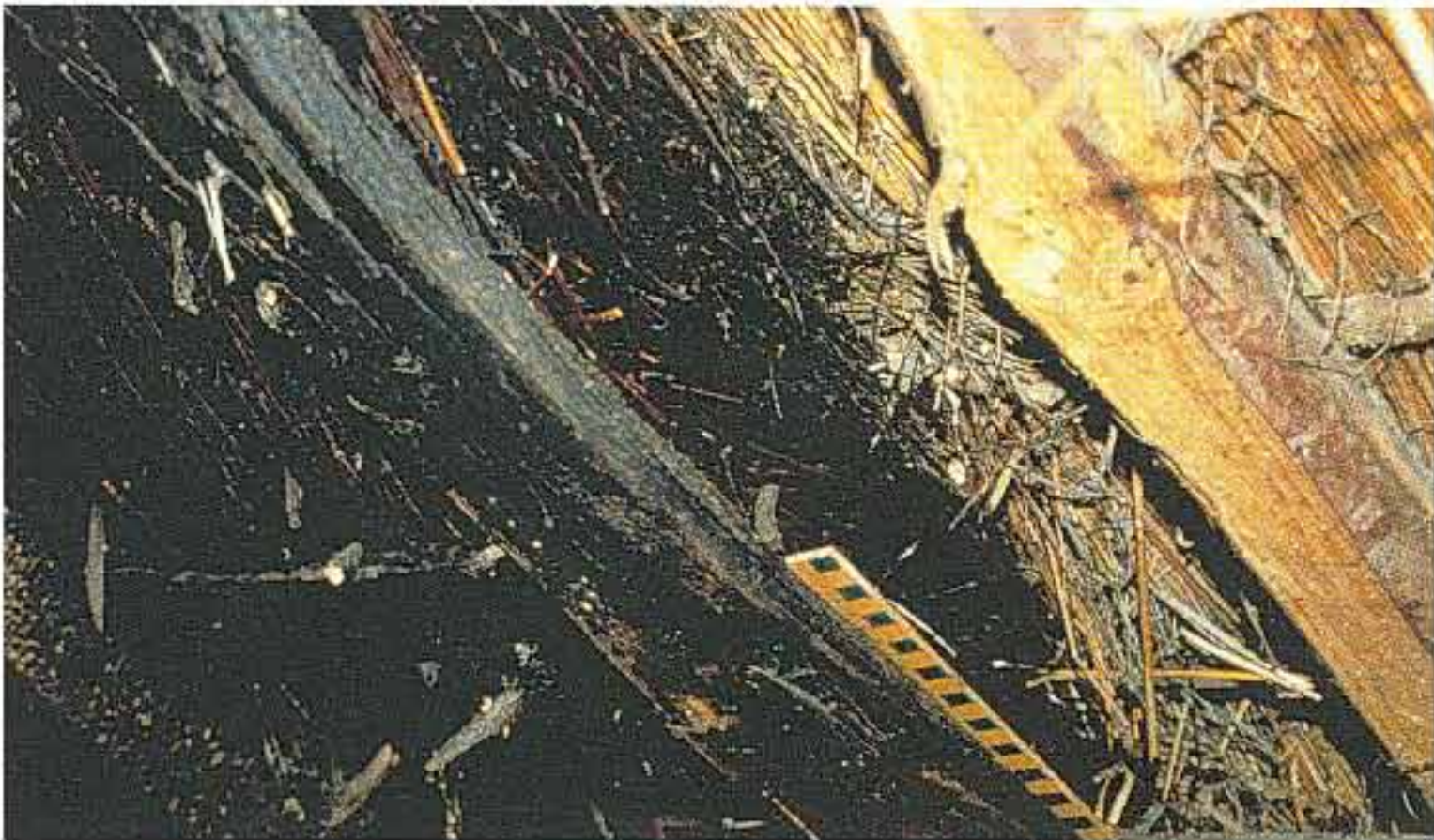
Fig 3 Smoke-blackened roofspace. In this photograph the contrast is clear between the sooting of the earlier portion of the roofspace (left), and the later part (right) which was built after the house ceased to have an open fire. (Photograph copyright © John B Letts)
