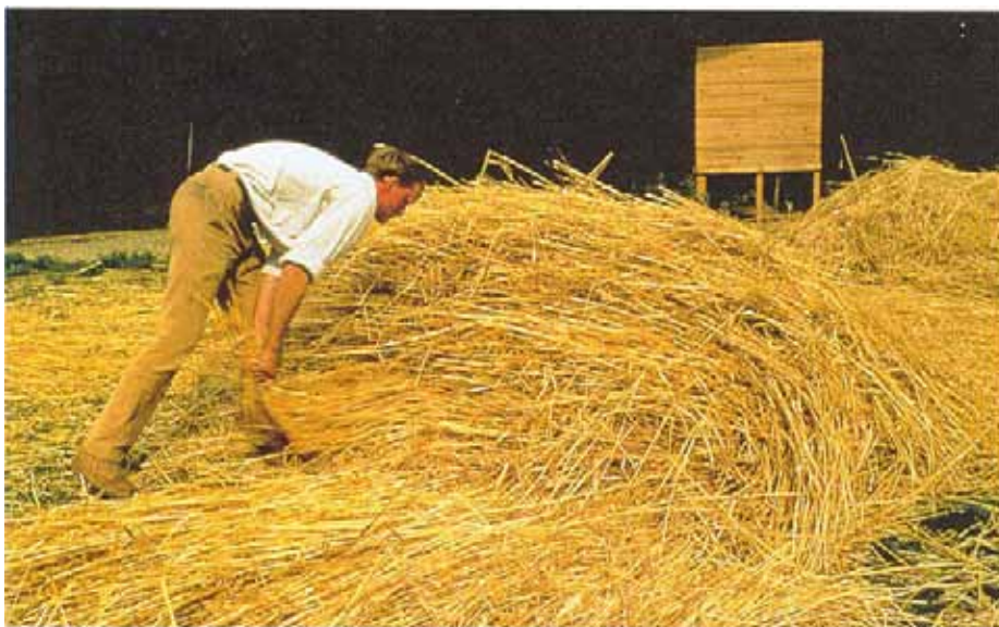
Fig 13 Drawing straw (Photograph copyright @ John B Letts)
