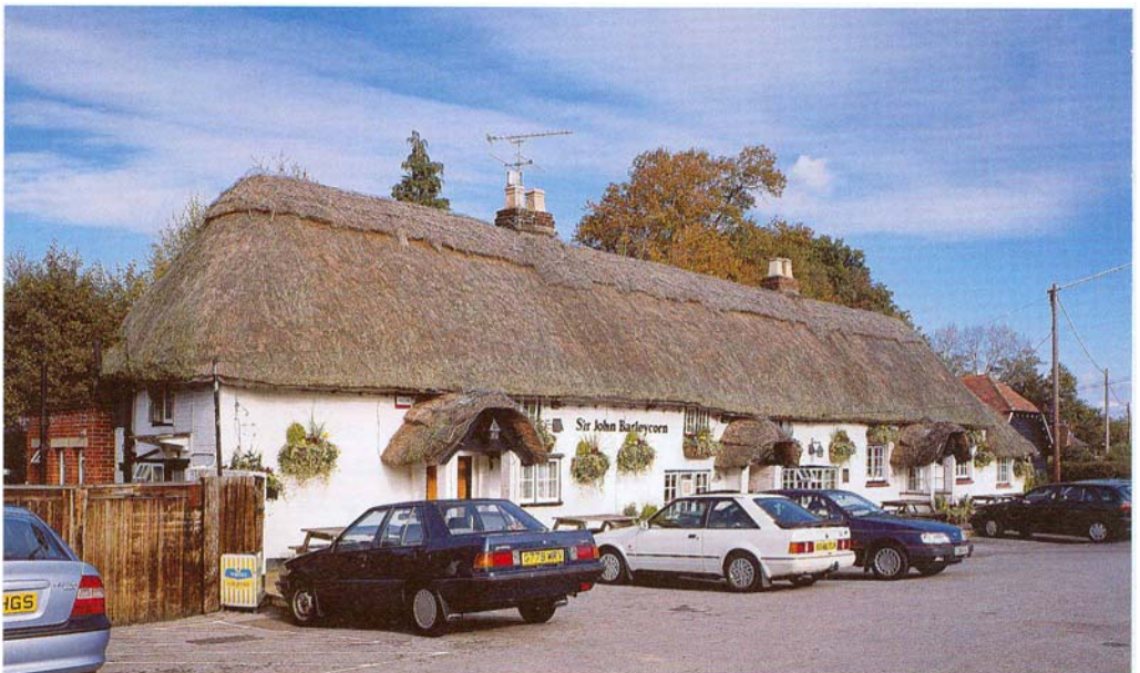
Fig 23 The Sir John Barleycorn, roofed in combed wheat reed with block ridge, in 1999
