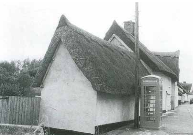
Fig 4 This long straw roof in Suffolk, with its distinctive wrapped and cut gables, is typical of the steep pitches found in east Anglia. (Photograph copyright @ Rural Development Commission)
