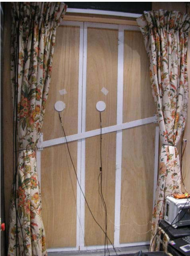
Figure 6: Insulating shutters installed
