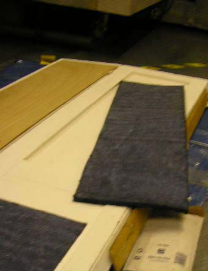
Figure 5: Insulating shutter panels
