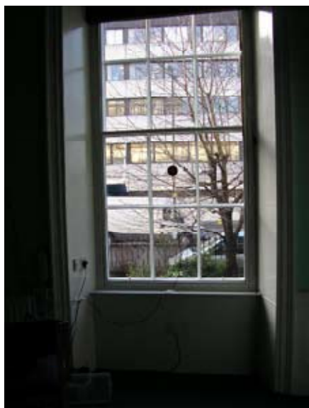
Figure 21: Heat flux sensor mounted on glazing of window in offices of Lister Housing Co-op, Lauriston Place, Edinburgh
