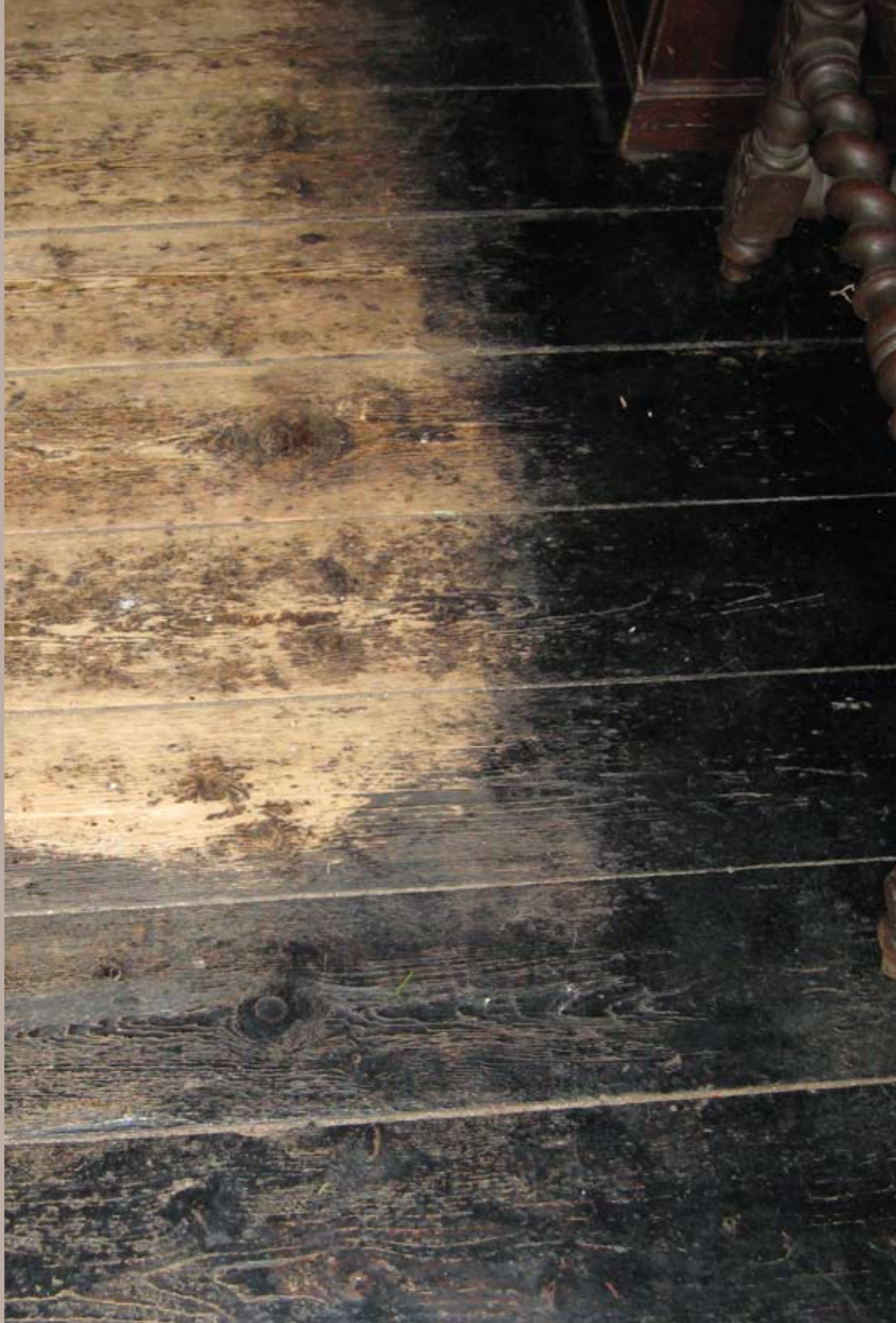
Mid 19th C timber floor, showing black painted boards and unfinished centre
