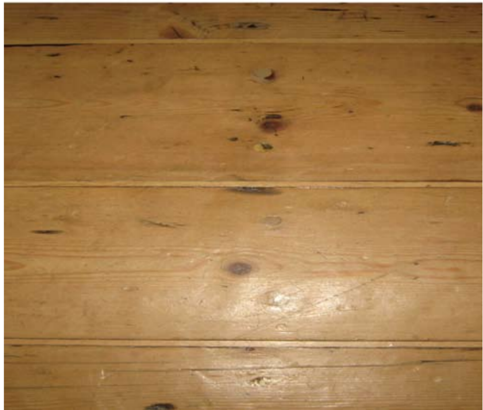
Softwood strips inserted where gaps are continuous
