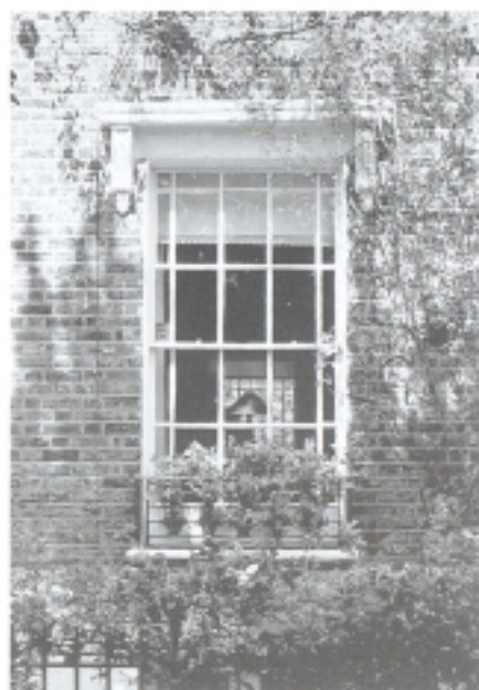
Wooden sash of the mid 1830s with decorative margin lights
