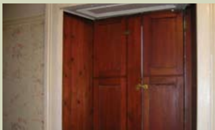
A mid 19th century shutter with original stain varnish on rear faces
