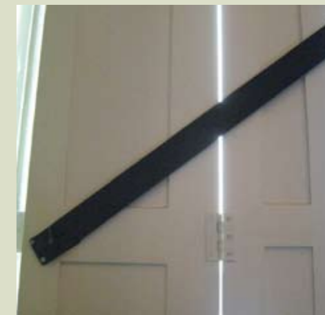
Shutters with a new stay bar in place
