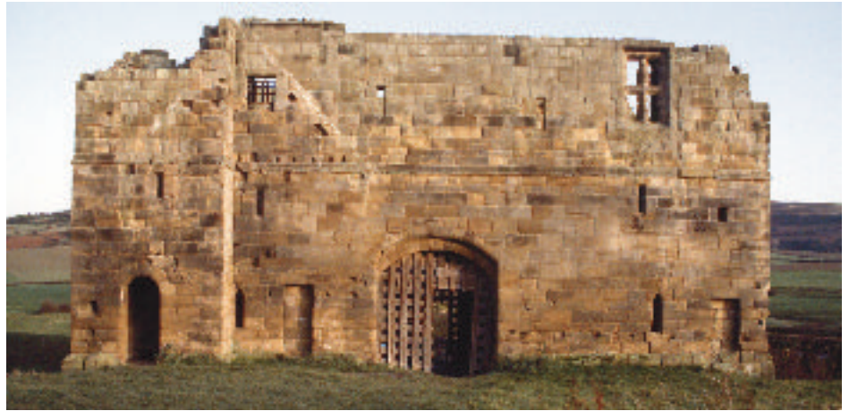
Figure 10 Where the view of an elevation is unimpeded an elevational photograph, taken in good light, may make an elevational drawing superfluous. (Whorlton Castle, Whorlton, N Yorks)
