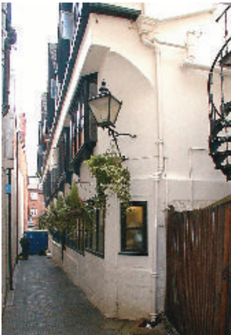
Figure 9 Site constraints may make it impossible to render elevational information photographically, and in such cases a drawn record might be considered. (130a High St, Oxford)
