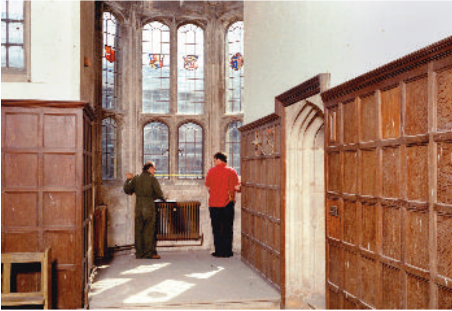
Figure 12 Traditional hand-surveying methods are necessary even where electronic equipment is available. With care they can produce highly accurate results in all but the most difficult conditions. (Apethorpe Hall, Apethorpe, Northants; AA044522)
